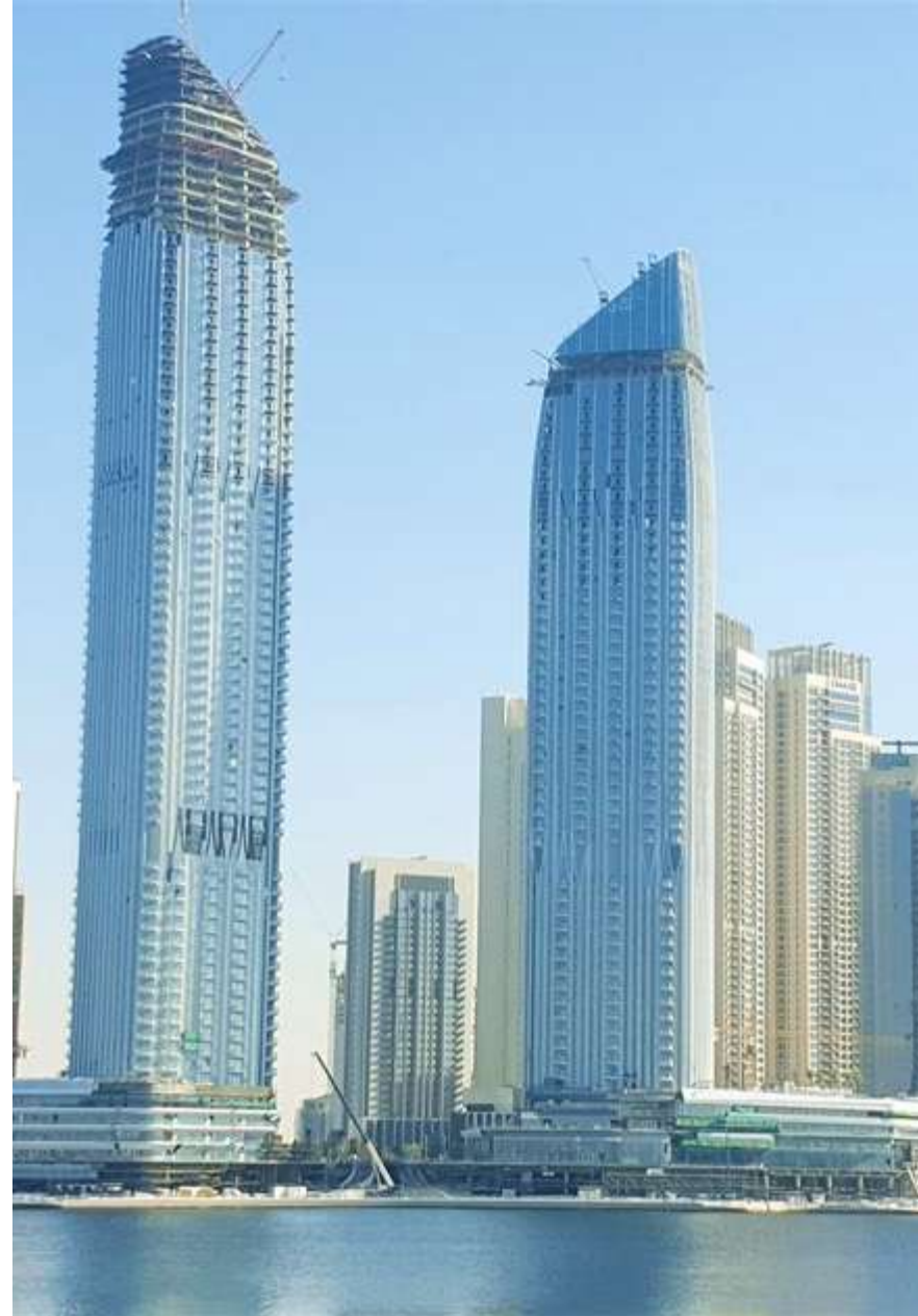
SITE PROGRESS – JANUARY 2022
