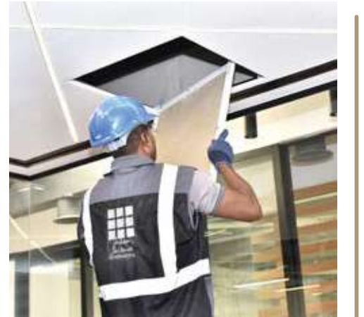
Plain Gypsum Ceiling
