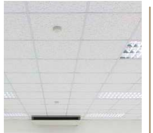
Gypsum Grid Ceiling
