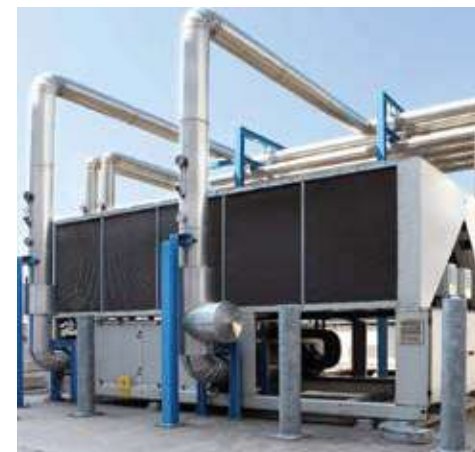
AHU's, FAHU's & VAV's
