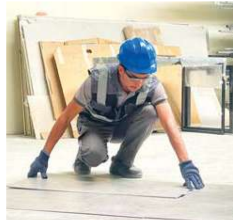
Floor and Wall Tiling
