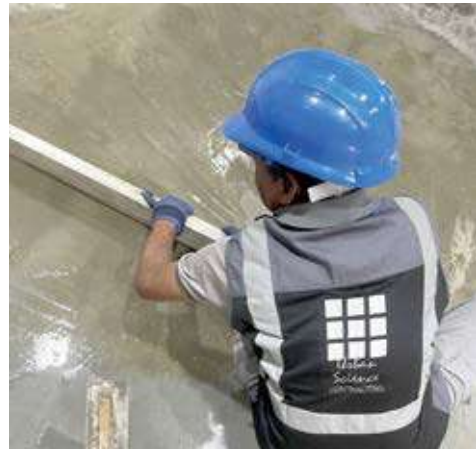
Floor Levelling / Cementing
